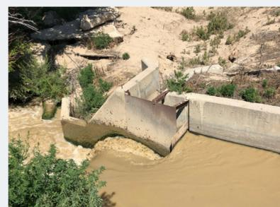
3) Depending on whether a utility decides to take water, the box divider channels water either to the irrigator's field, or the utility's water treatment facility ("2017 Annual Report", 2018).
