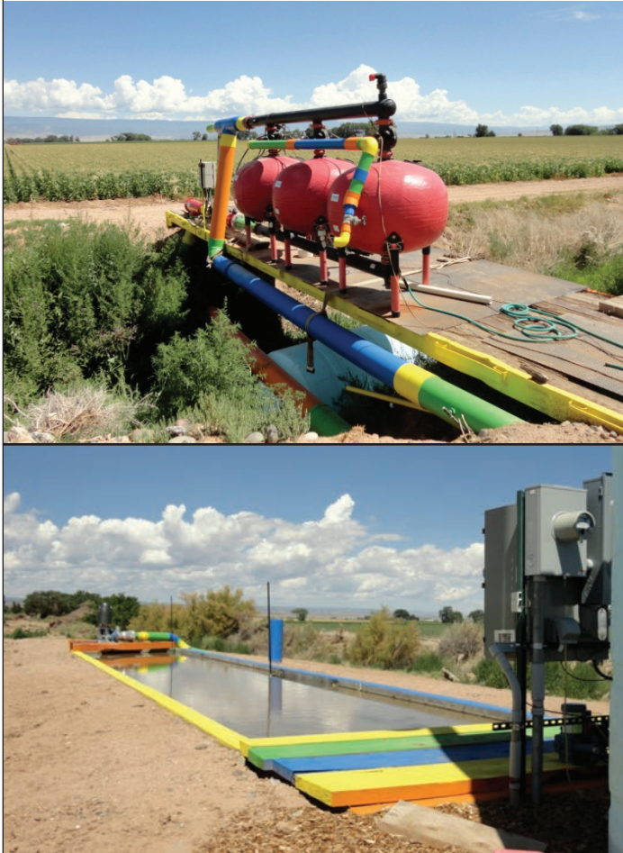
Figure 6: State-of-the-art Subsurface Drip Irrigation System and Settling Pond
