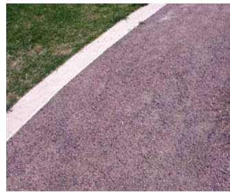
B Stabilized Aggregate
