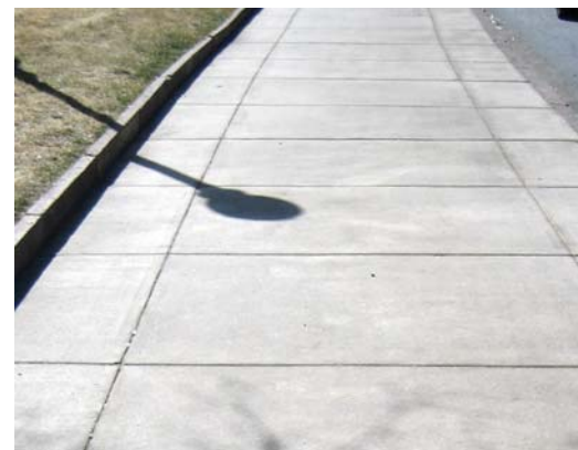
A Concrete with 1' Band
