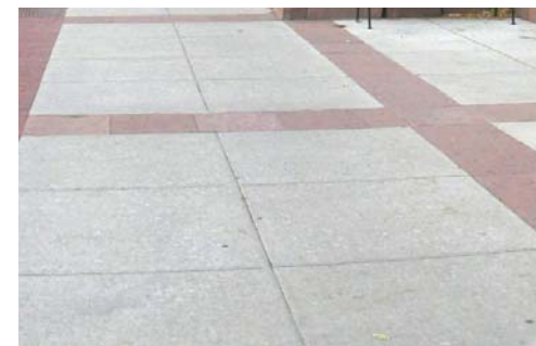
Concrete with Interval Stone Banding
