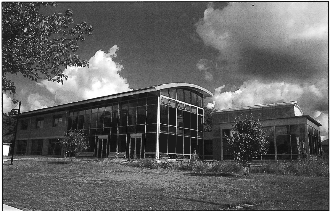
A 60 kW grid-connected photovoltaic array on the roof of Oberlin College's Adam Joseph Lewis Center for Environmental Studies generates a substantial portion of the annual electricity use of the facility.
