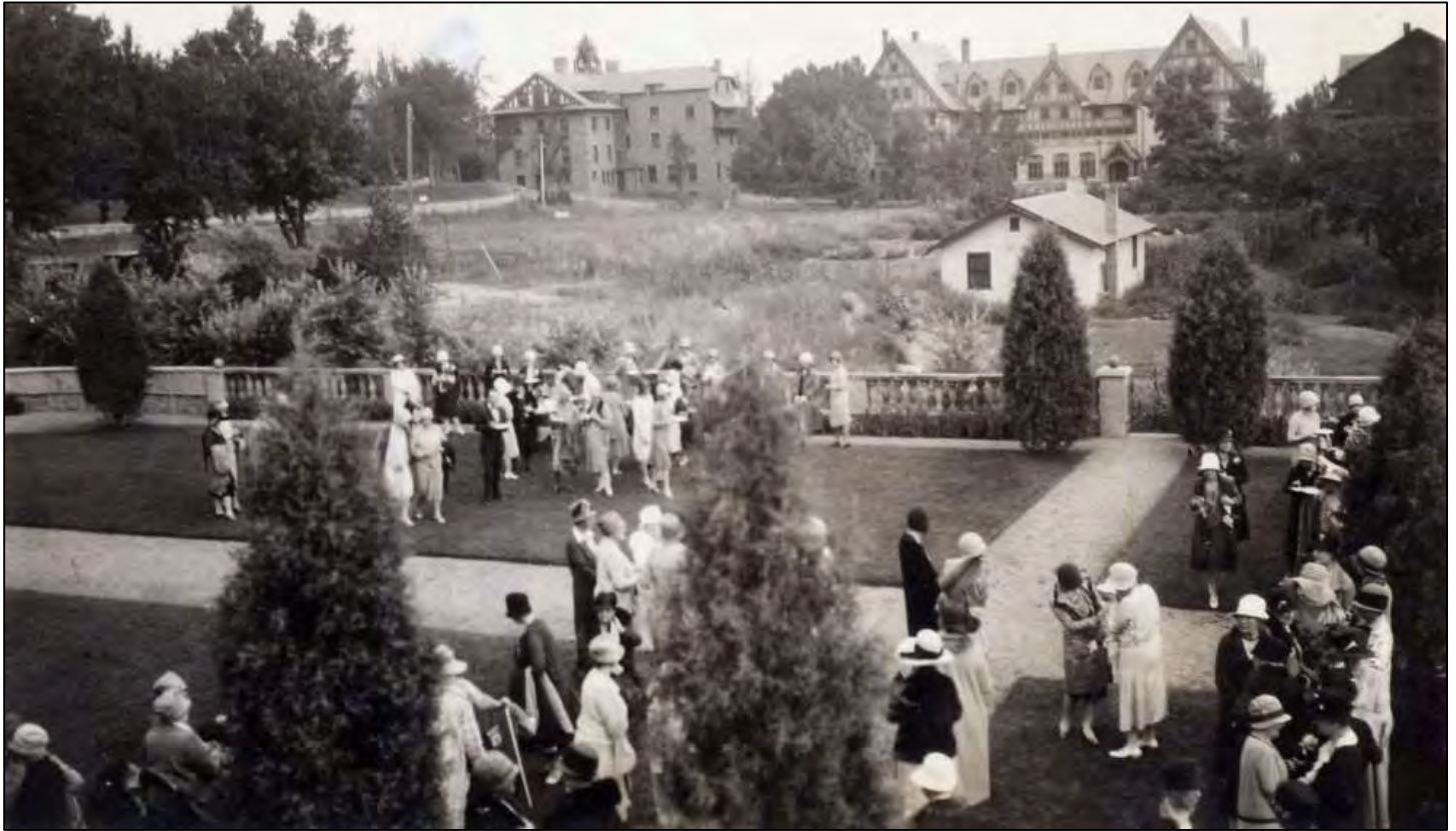
Figure 4. A late-1920s or early-1930s view south-southeast documents a garden party underway in the sunken lawn south of the house. Two main gravel paths form a cruciform design and narrower gravel paths are present along the balustrade. Buildings of Colorado College are visible in the distance. Courtesy of Tor Hylbom, photographic collection, Arcadia, California.
