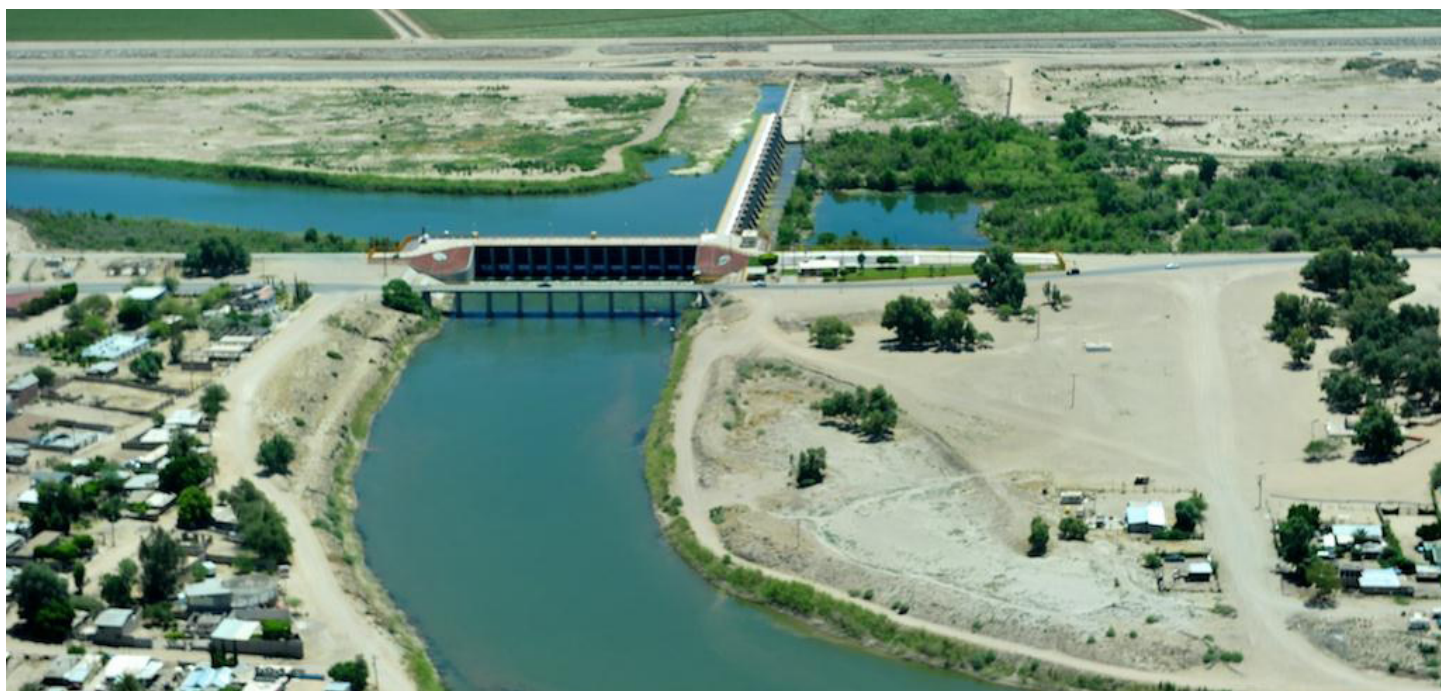
Thomas McMurray, Aerial Photograph of Morelos Dam
