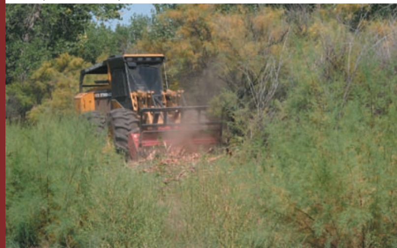
This bulldozer is equipped with a HydroAx to mow down woody invaders. Removing invasives at this site in Florence, Colorado, will not be enough. Active revegetation is likely needed. Photo by Anna Sher.
