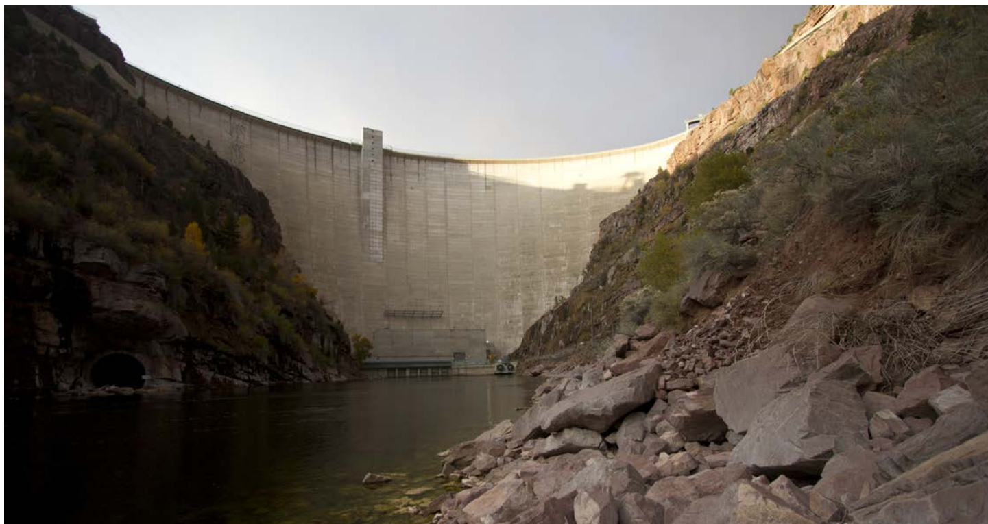
Will Stauffer-Norris, Flaming Gorge Dam
