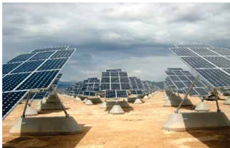
Solar Array at Nellis Air Force Base near Las Vegas, Nevada
