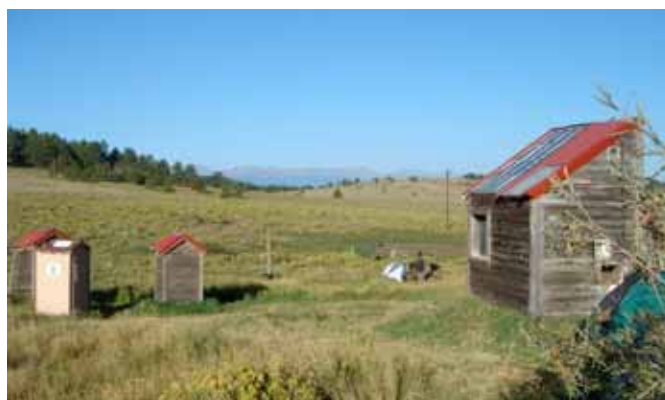
Huts with Solar Panels, Bear Basin Ranch, Westcliffe, Colorado
