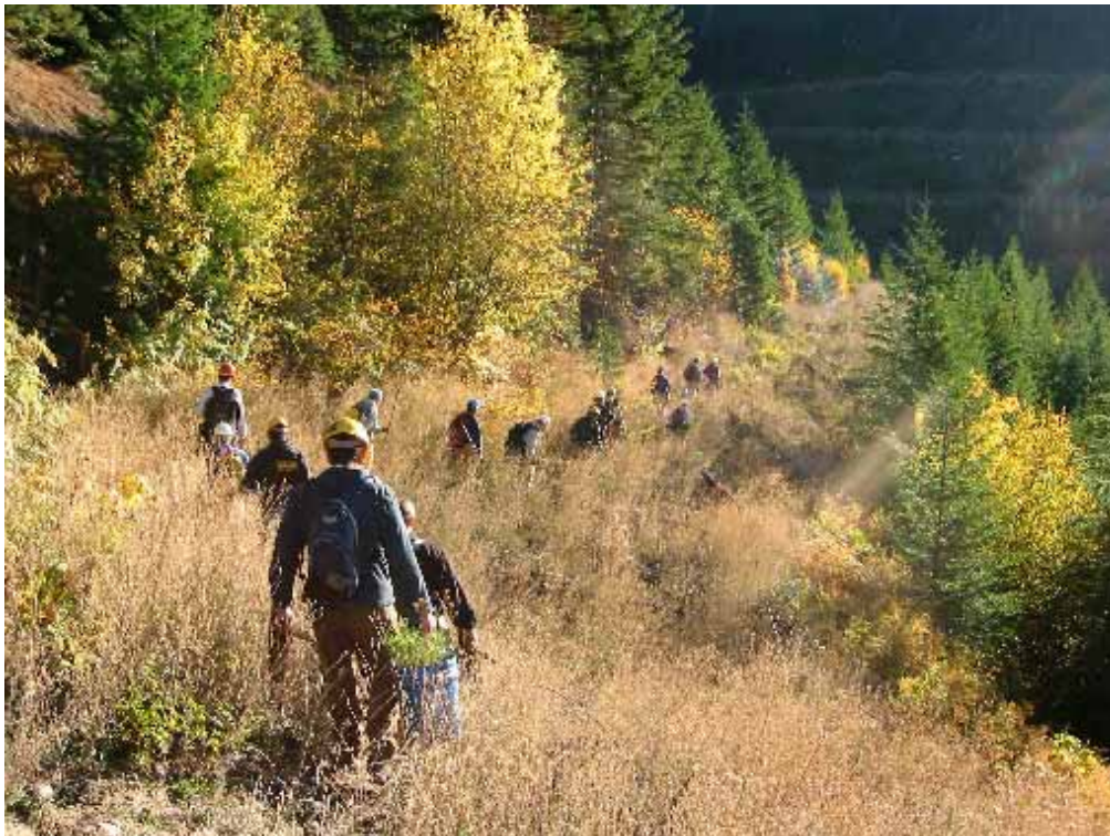
Montana Conservation Corps revegetating removed road
