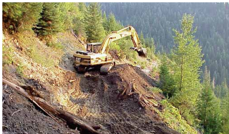
Road Removal in the Clearwater National Forest, Montana
