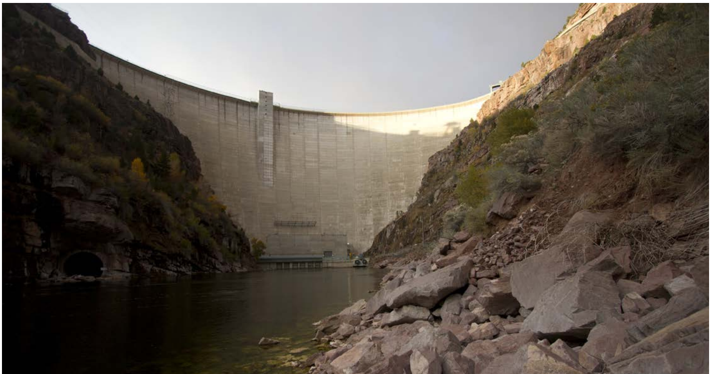
Will Stauffer-Norris, Flaming Gorge Dam
