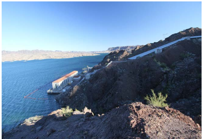
Lake Havasu and the pumping station for the Colorado River Aqueduct
