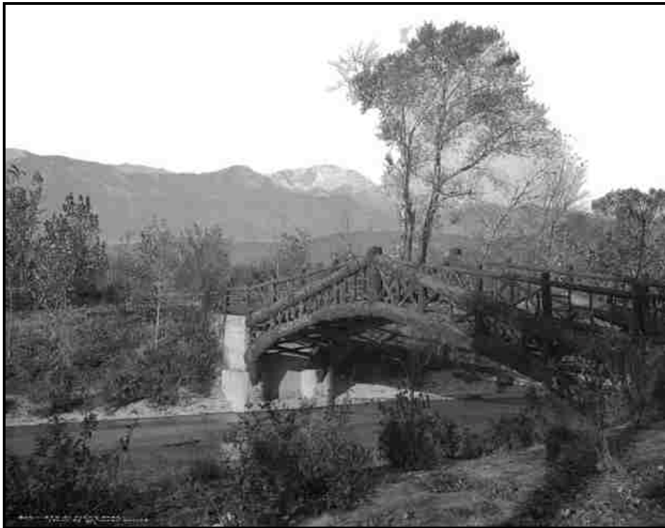
Figure 2. The original construction of the park ripped the banks of Monument Creek, but the channel was still sufficiently narrow to be spanned with this Rustic bridge of unpeeled logs. SOURCE: Denver Public Library, Western History and Genealogy Department, L.C. McClure image number MCC-809, Denver, Colorado.
